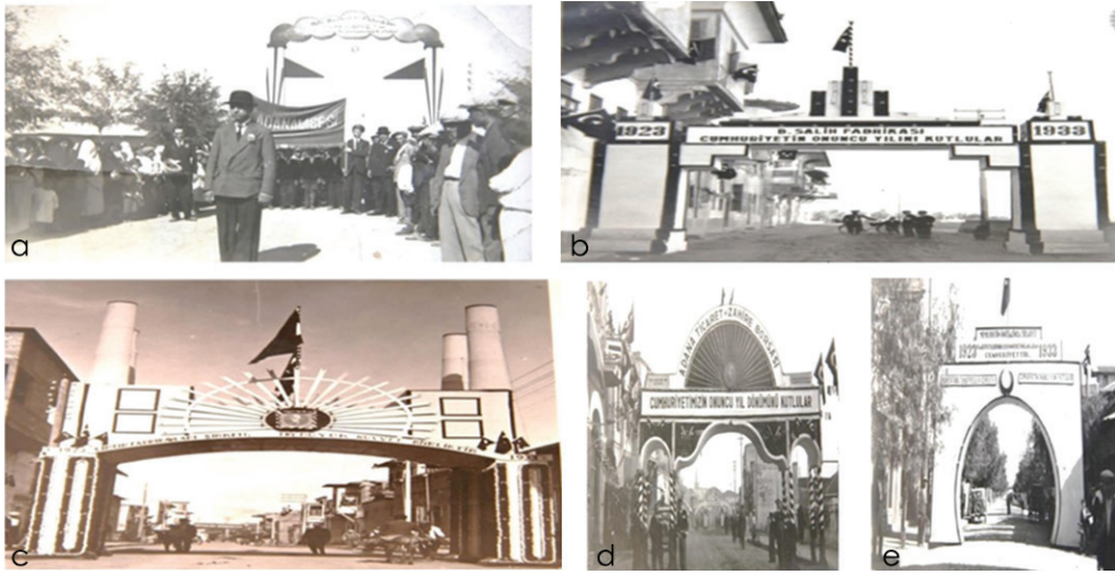
Figure 6. a) Tak of Millî Mensucat Factory, b) Tak of Şalih Factory, c) Tak of Çırçır Factory, d) Tak of the Chamber of Commerce and Grain Exchange, e) Tak of the Haberdashers' and Drapers' Association (Kalafat & Kalafat, 2022), Adana 1933.
