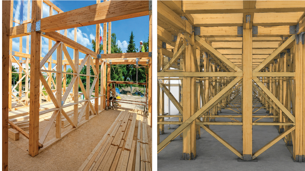
Figure 4. Wall frame of the Osmaniye Timber Housing Project (Unpublished company working report, 2023, NASWOOD).
