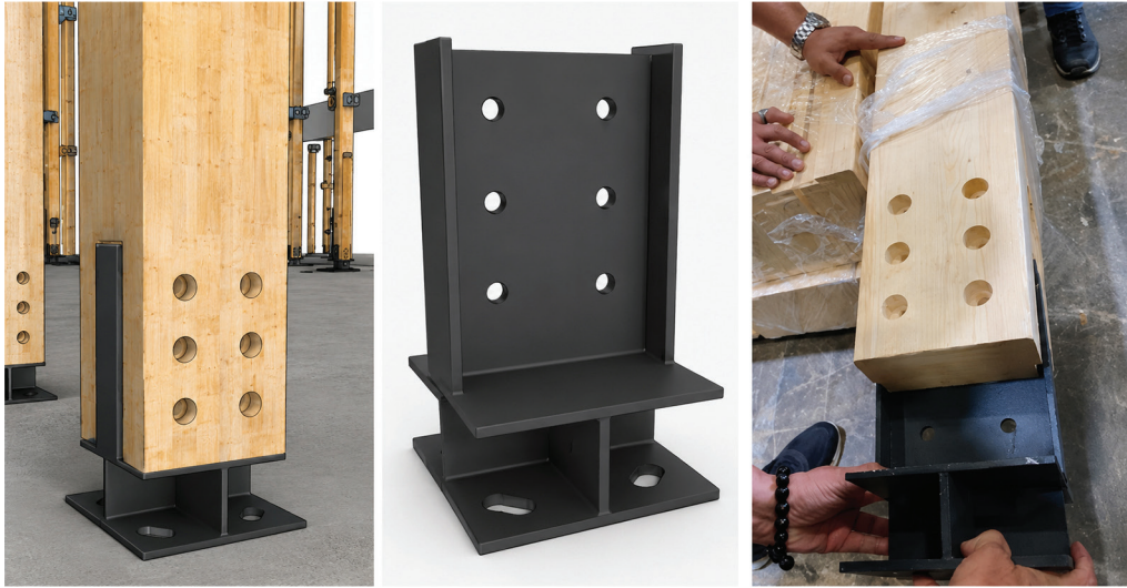
Figure 5. Column anchorage connection of the Osmaniye Timber Housing Project (Unpublished company working report, 2023, NASWOOD).
